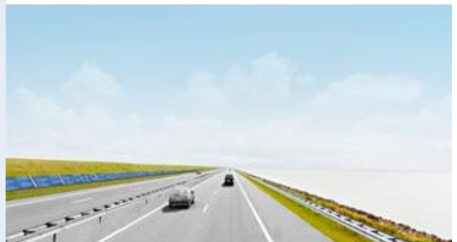
Solar power plant over 24 km
